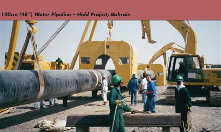
120cm (48") Water Pipeline - Hidd Project, Bahrain
