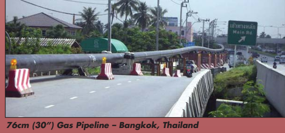
76cm (30") Gas Pipeline - Bangkok, Thailand
