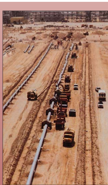
76cm (30") Gas Pipeline - Haradh Project, Saudi Arabia
