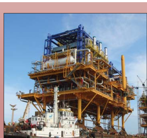
Welding Steam Line - Slattery Project, NYC
