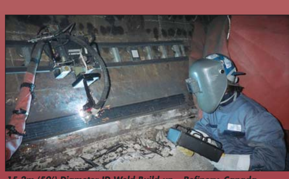
15.2m (50') Diameter ID Weld Build-up - Refinery, Canada
