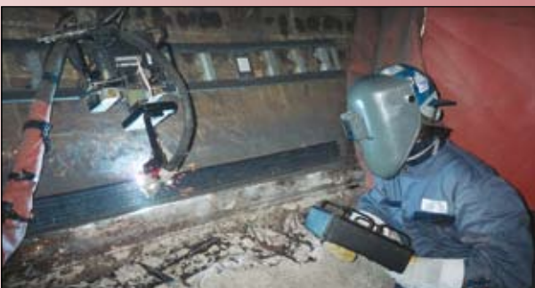
15.2m (50') Diameter ID Weld Build-up - Refinery, Canada
