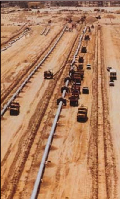
76cm (30") Gas Pipeline - Haradh Project, Saudi Arabia
