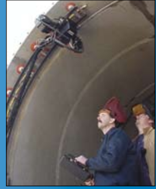
Pipeliner mounted on Flx-Track in 3.3m (11 ft.) diameter stainless steel duct
