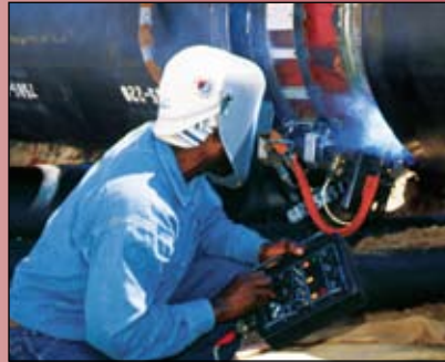
Welding Steam Line - Slattery Project, NYC
