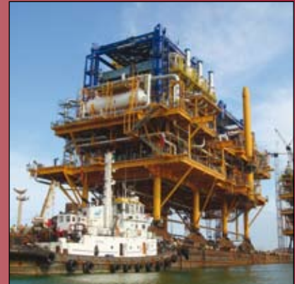
Offshore Platform Topside Module - Swecomex Project, Mexico
