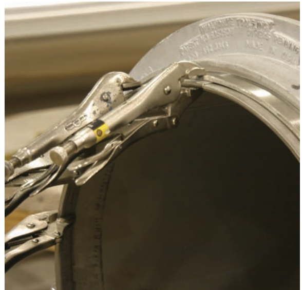
Installing the backing ring to a section of stainless sheathing.
