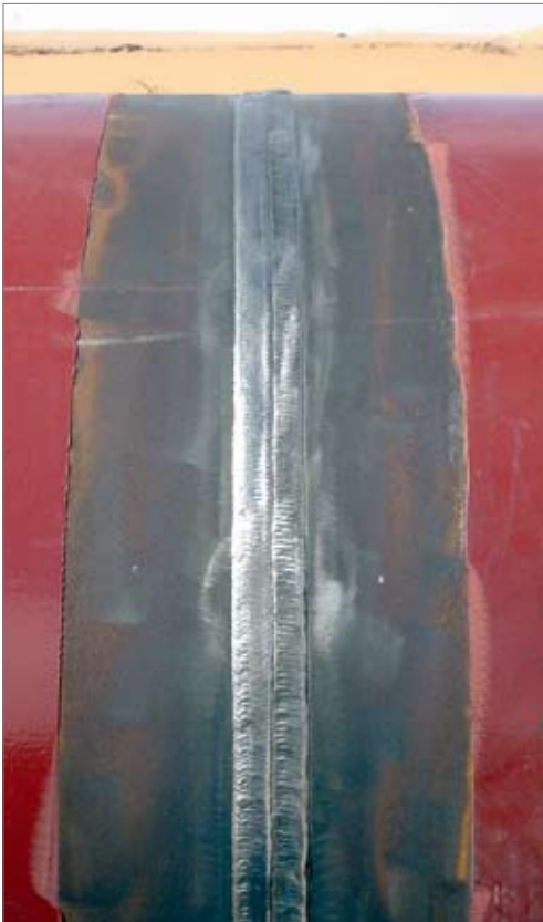
Figure 4. Typical weld appearance of a mechanised welded joint.
