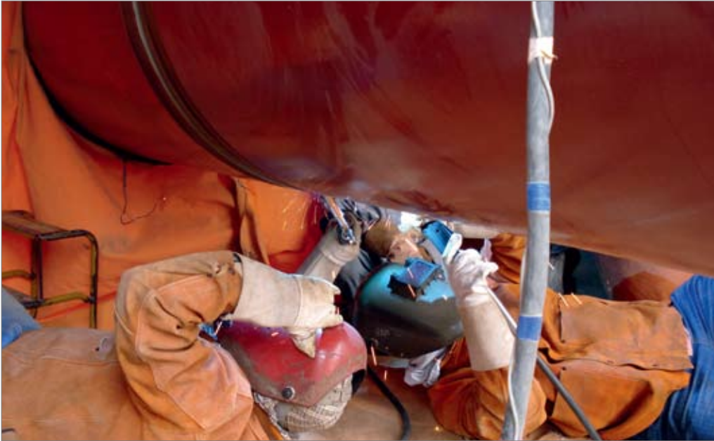
Figure 2. STT root pass welding
