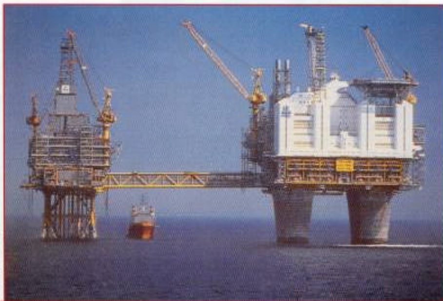
Norwegian offshore platform, one of several structures to benefit from the use of orbital welding.
